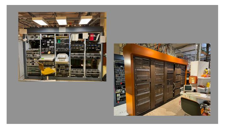
On our second floor, we have our computer-controlled (#3 ESS) and fully digital switches (Nortel DMS-10).
